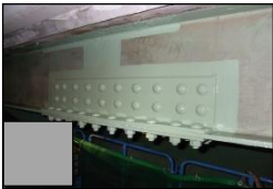
(b) patch plate repair
