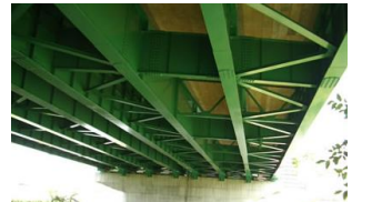
Fig.1 Members of plate-girder bridge
