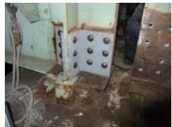
Fig. 2. Repair with Steel Plates
