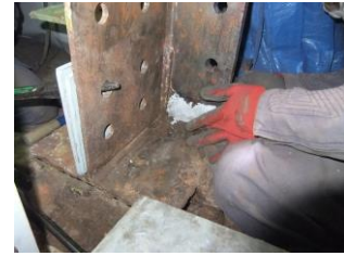
Filled with Adhesive
